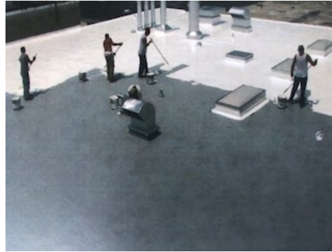
Hood Roof Restoration
